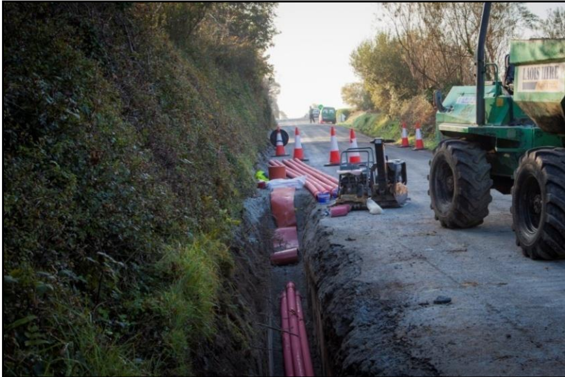
Figure 3-4 Typical duct installation works for a grid connection cable trench
