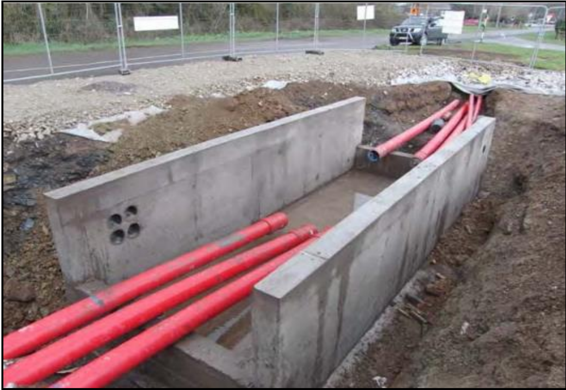
Figure 3-8 Typical Joint Bay Construction
