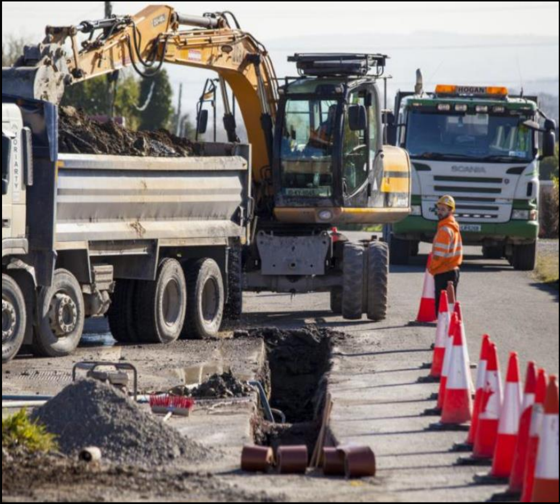
Figure 3-3 Typical excavation works for a grid connection cable trench
