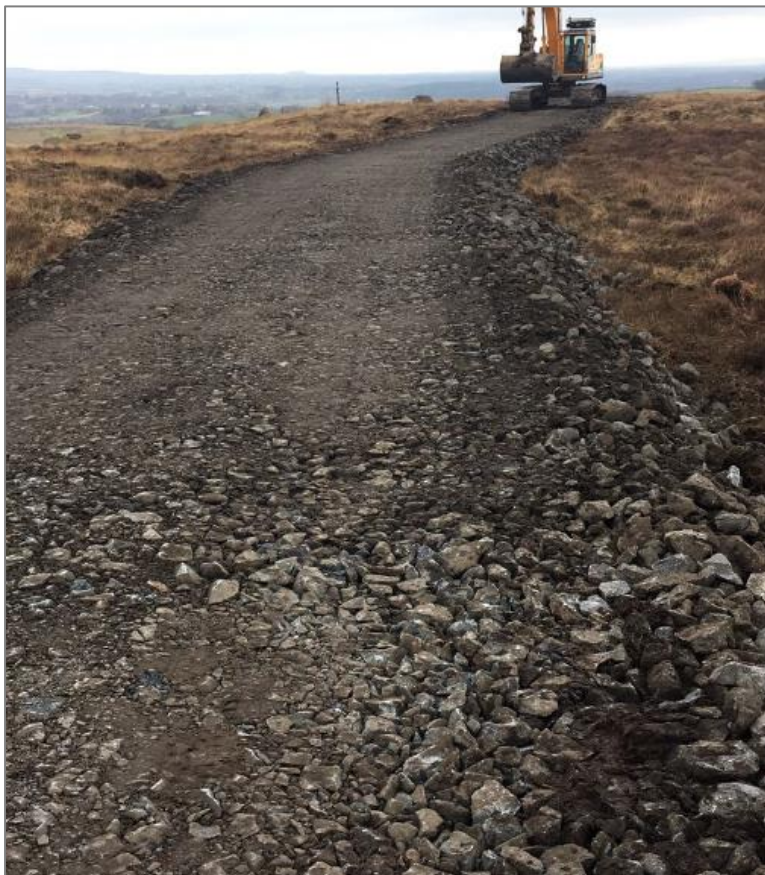
Figure 3-2 Typical Access Road fully instated
