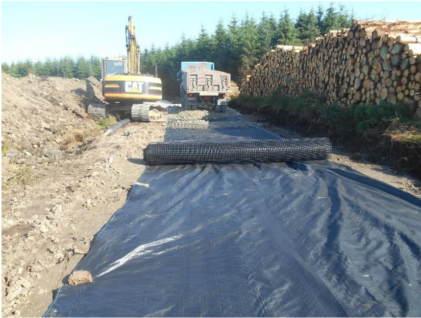
Figure 3-1 Crushed Rock Roadway Build-up with Geotextile
