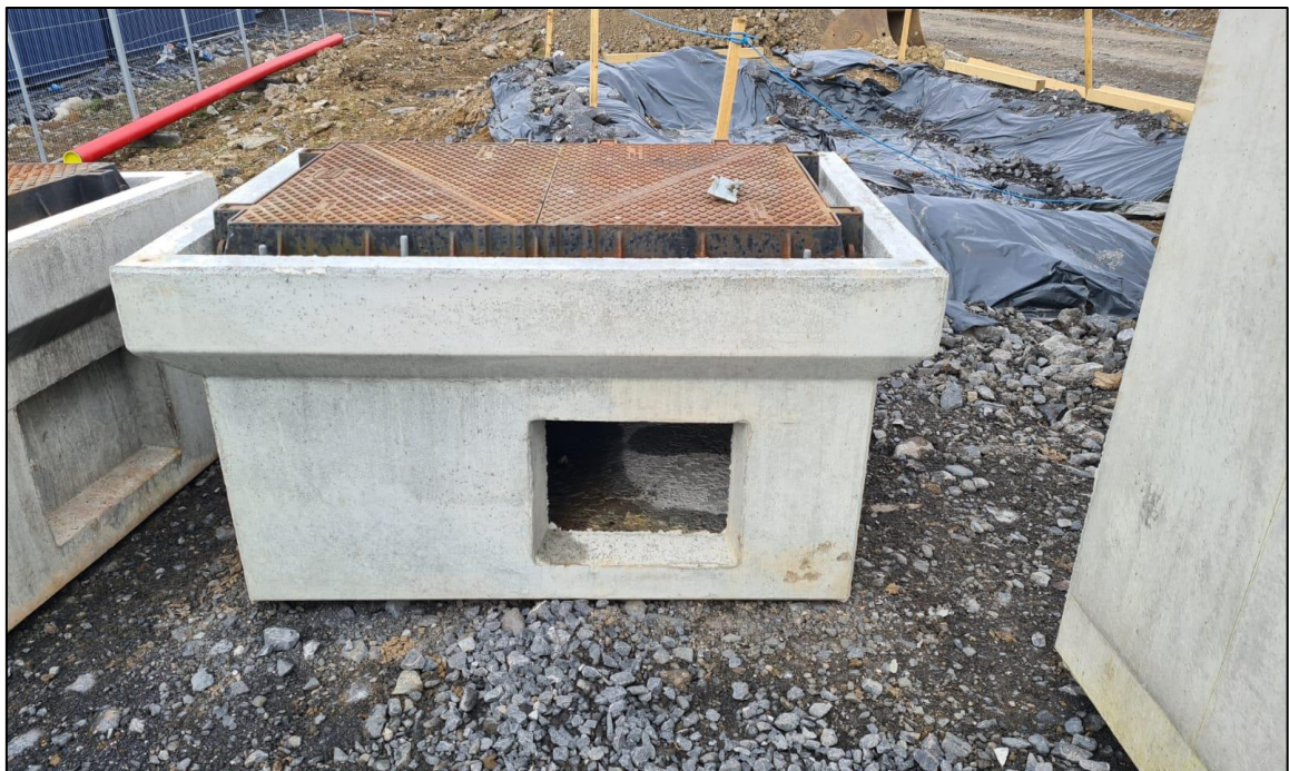
Figure 3-9 Typical Earth Sheet Link Box Construction
