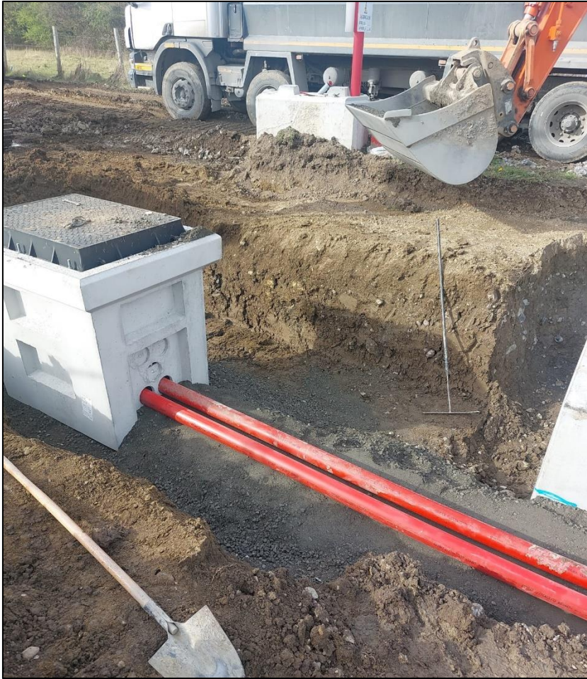
Figure 3-10 Typical Communications Chamber Construction
