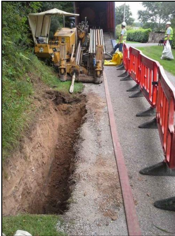
Figure 3-6 Typical directional drilling rig and launch pit
